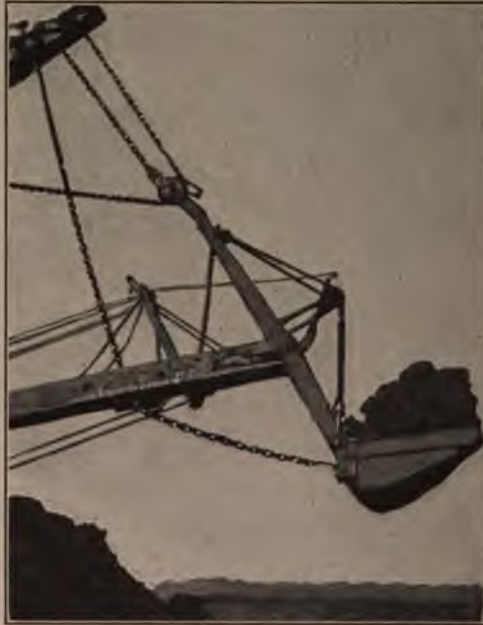
Dipper and Dipper-arm of Walking Dredge.
